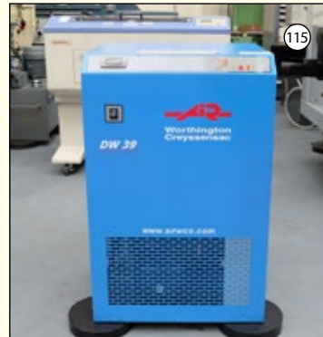
WORTHINGTON CREYSENSAC Type DW39: Water Chiller. Refrigerment R404A. Power 1KW. Single Phase 230v.
